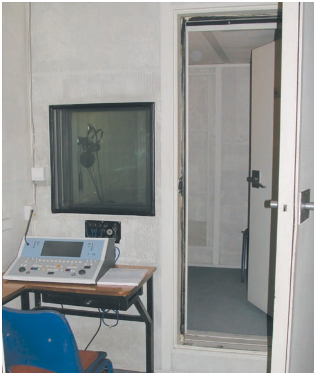
Fig. 1.2.4 Soundproof hearing test rooms
